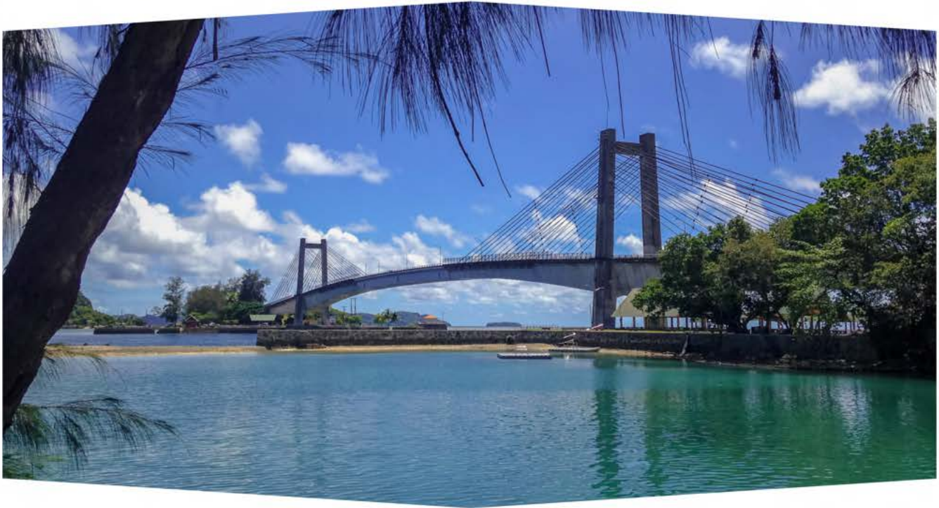
Japan-Palau Friendship Bridge, which connects Koror and Airai Source: Adobe Stock Images, Kaori
