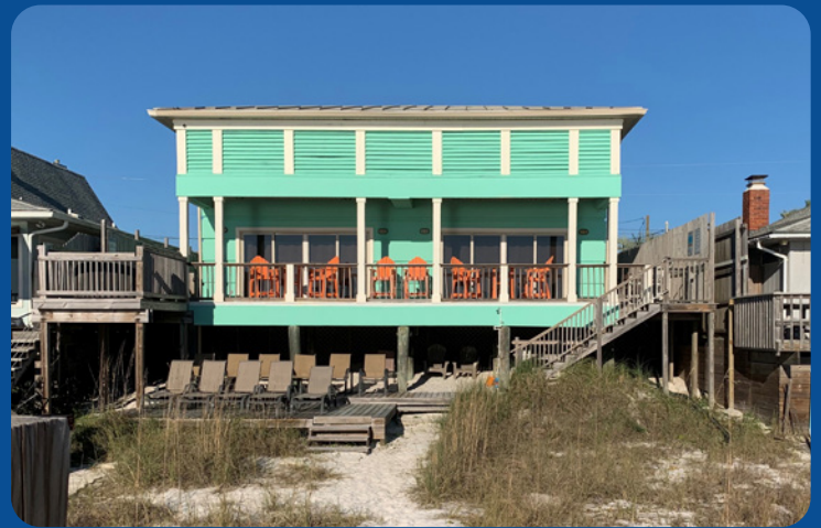
Structure elevation to mitigate flood damage
